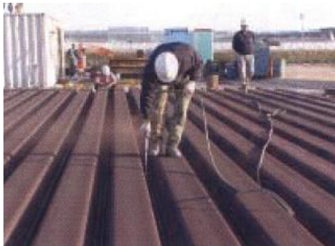
Cleaning of sheet piles interlock joints
