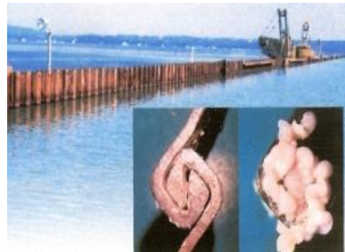
Expansal* Interlock expand in presence of moisture
